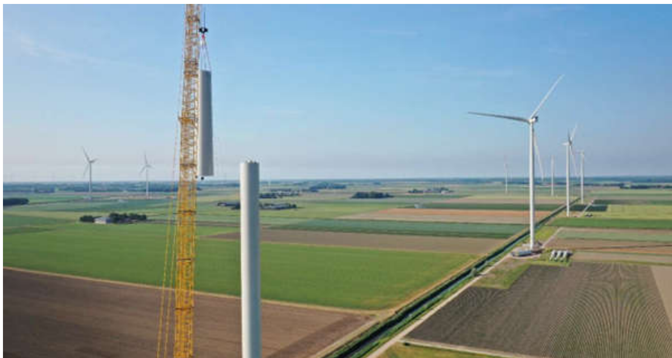
Windfarm Olsterwind wind turbines being constructed.
